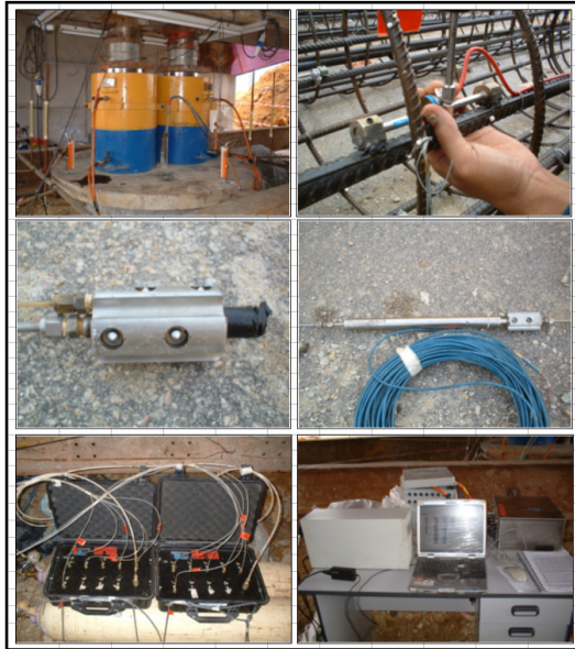
Fig.2: Typical pile test instrumentation and monitoring set-up
